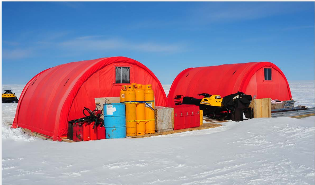
NEW SWISS CAMP STATIONS, REBUILT AFTER THE PLATFORM COLLAPSED DUE TO SURFACE MELTING. WOODEN PLATFORM WITH 16 WOODEN LEGS DRILLED 8 M INTO THE ICE.
